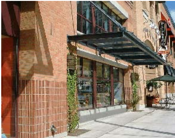
This building illustrates thicker walls at the base and the use of high-quality materials.
