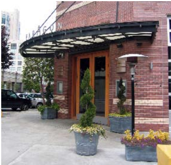
Proper corner treatments provide a clear view and enhance the public realm while adding architectural interest in design
