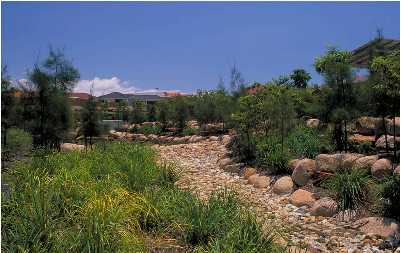
The deployment of BMPs on a site can take many forms, which allows the facilities to integrate with landscaping while still providing optimal stormwater functionality. These examples show bioretention areas within an outdoor courtyard (above left), a vegetated swale and filter strip serving as a buffer for homes (above right), and a rocky swale area meant to be appealing while dry but able to handle infrequent large flows.
