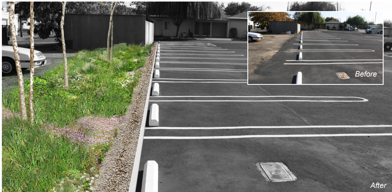
Filter strips can be as simple as a gentle slope in grass that receives runoff from an adjacent strip of parking stalls.
