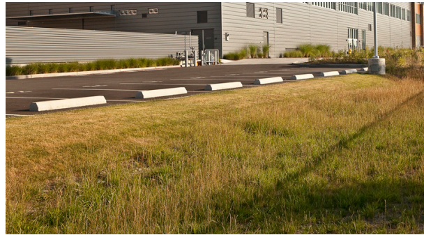
Filter strips can be as simple as a gentle slope in grass that receives runoff from an adjacent strip of parking stalls.
