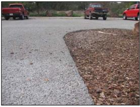
modular blocks (stone or concrete blocks interspersed with pervious material such as gravel or sand), granular pavement (crushed aggregrate with wood mulch and cobbles), porous asphalt, and pervious concrete.
