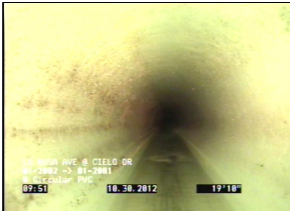
Figure 6.4 – Example of Pipe in Good Condition
