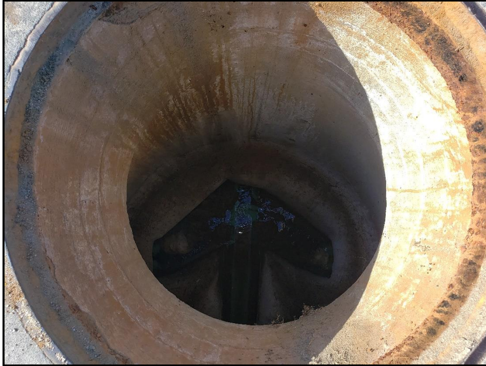
Figure 6.10 – Example of Manhole in Good Condition
