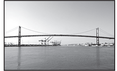
Vincent Thomas Bridge
