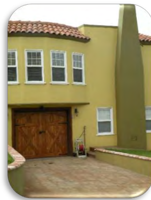
A remodeled historic single family home (top) and duplex units (bottom) in Colma's Sterling Park neighborhood.
