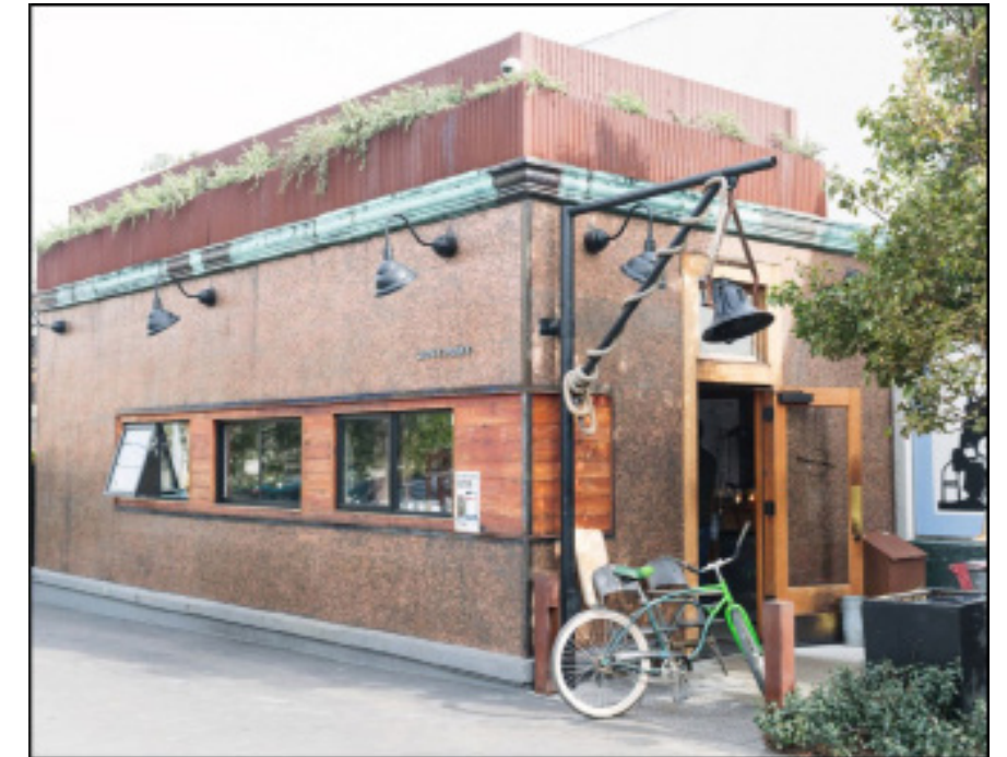
EXAMPLE OF ACCEPTABLE ADAPTIVE RE-USE
