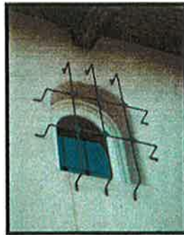
Wrought iron grill work over window
