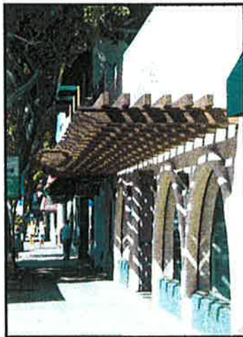
Wood trellis structure acts as an awning providing shade interest to facade.
