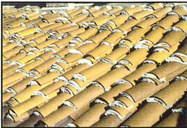
Grouted terra cotta tile roof
