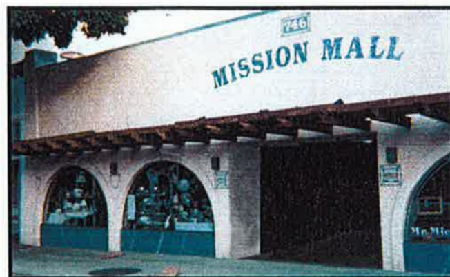
Trellis used along blank wall to accent entry and add interesting shade and shadow detail
