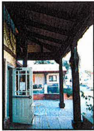
Existing covered walkway.
