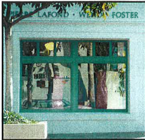
Storefront windows located on the first floor distinguish it as a publicly oriented space.
