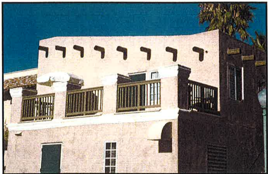
Balconies on upper floors are encouraged and help to break up large massing.
