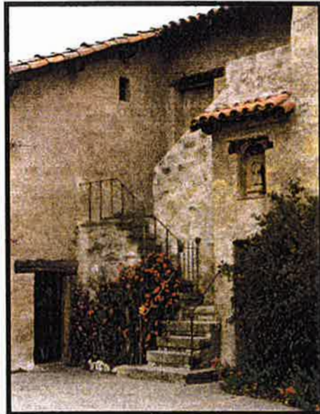
Stairway design should be integrated with the building's overall character and design.
