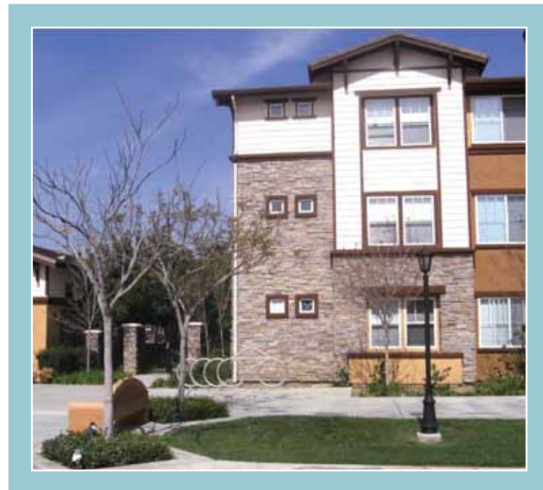
Use of varied facade articulation and materials.
