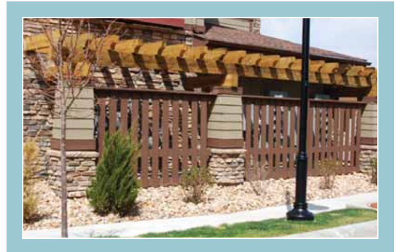
Screening of mechanical equipment
