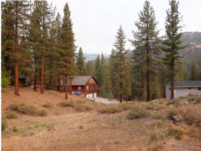
Lot overview, 002-392-020-0. View Northeast; Exp 301
