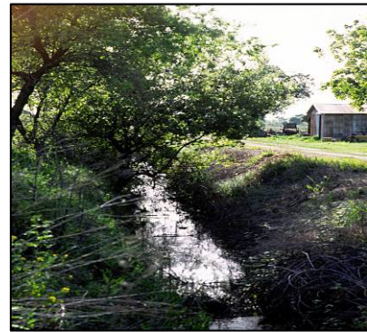
Exhibit Design-3. Agricultural Drainage Channel
