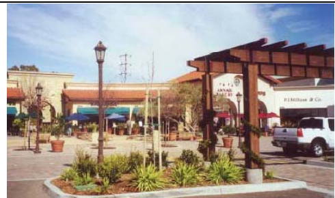
Exhibit Design-43. Parking Lot Shade Structure
