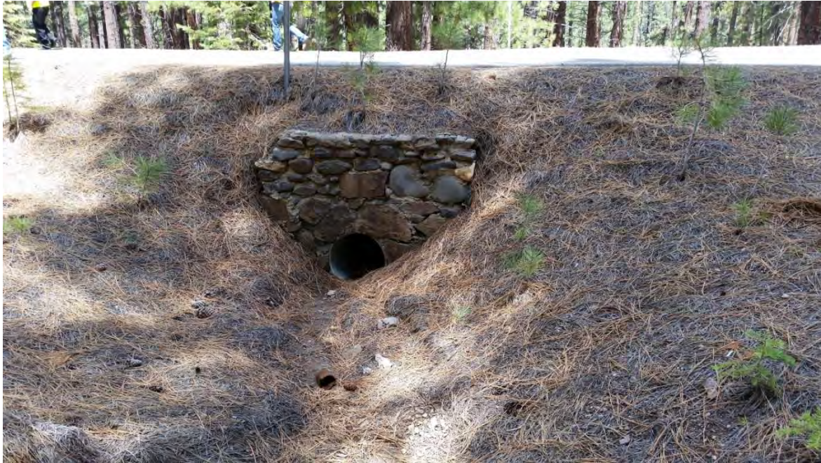
Stone-lined culvert headwall.
