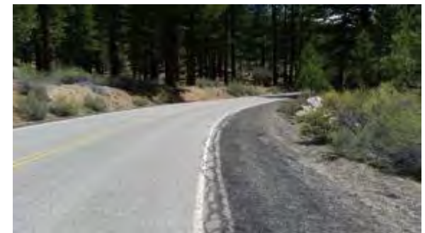
Photo 12. Example shoulder deterioration; Great Basin mixed scrub, and Jefferey pine forest communities, facing east.
