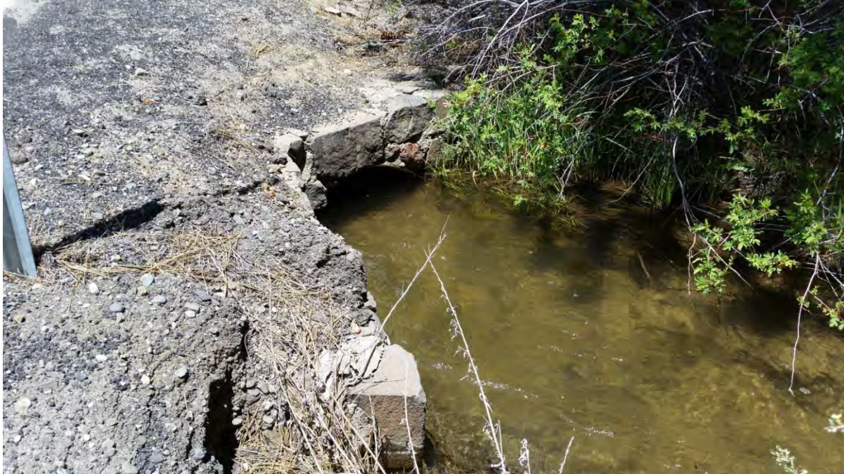
Town Ditch culvert entrance under Hot Springs Road
