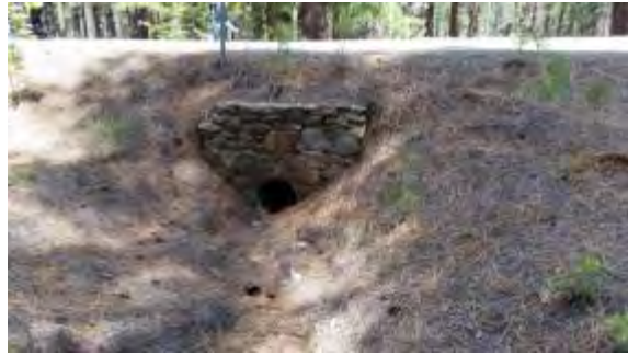
Photo 14. Existing culvert under Hot Springs Road, facing north.
