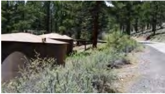
Photo 13. Markleeville Water Company water tanks located along Hot Springs Road, facing west.
