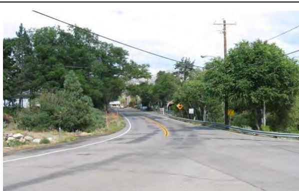
Photo 2. Hot Springs Road at its intersection with Laramie Street, facing east.
