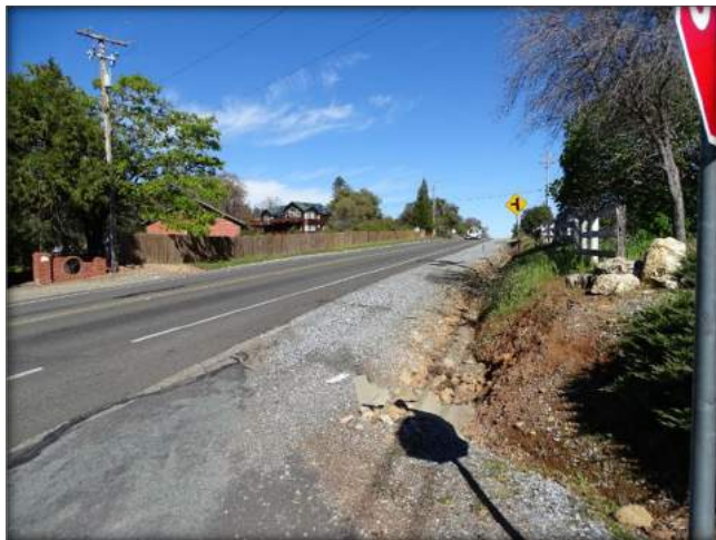
Sight distance at the intersection is limited by a crest vertical curve on Ridge Road, east of the intersection. The maximum sight distance to the east is 575'. Advance intersection warning signs are posted at this location and there is a street light at the intersection. There is no turn lane on Ridge Road on to Running Gold Road, therefore, though traffic on Ridge Road must stop behind the turning vehicle.
