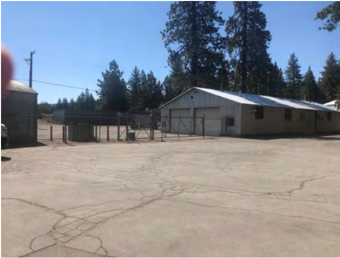
Vehicle storage yard.
