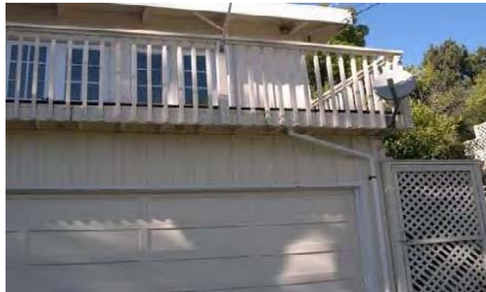
The figure above shows wood deck, built on wood 2x6 'sleepers' on a solid surface deck (above a garage).
