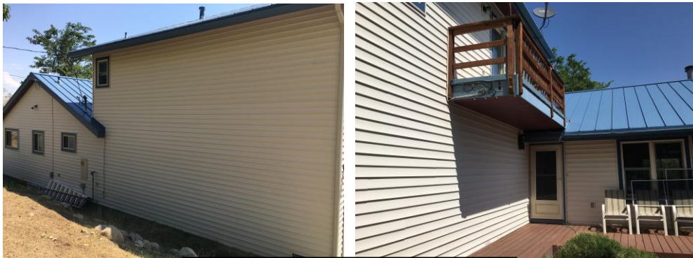
Fire resistant roofing and siding
