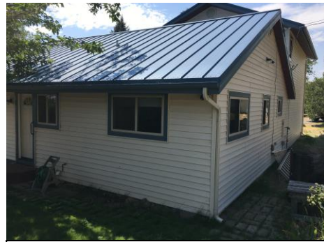
Plants clear of building corners
