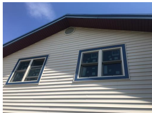
Enclosed eaves/secure vents
