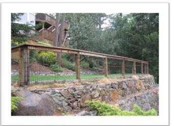
addition to soil, shall be designed in accordance with accepted engineering practice to ensure stability against overturning, sliding, excessive foundation pressure, and water uplift. Retaining walls shall be designed for a safety factor of 1.5 against lateral sliding and overturning. This section shall not apply to foundation walls supporting buildings."
